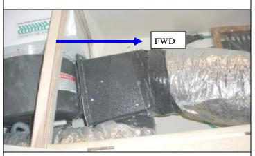
Install this air duct then run it forward thru main bulkhead cutout then temporary store the air duct for further installation.
