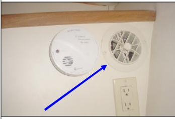
Mount and secure air vent on Aft cabin hanging locker aft face.
