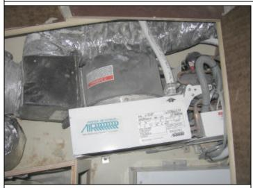
Install AC discharge hose, use 2 designated hose clamps to hold this hose. Ensure there is no obstacle around the fitting before you install this hose.
