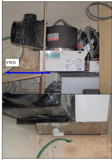
Drain elbow facing inboard, install drain hose on this elbow, then run the hose down in bilge.
