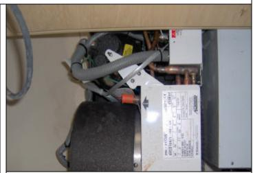
AC discharge hose will be installed in engine stage, ensure the fitting cap is on the fitting.
