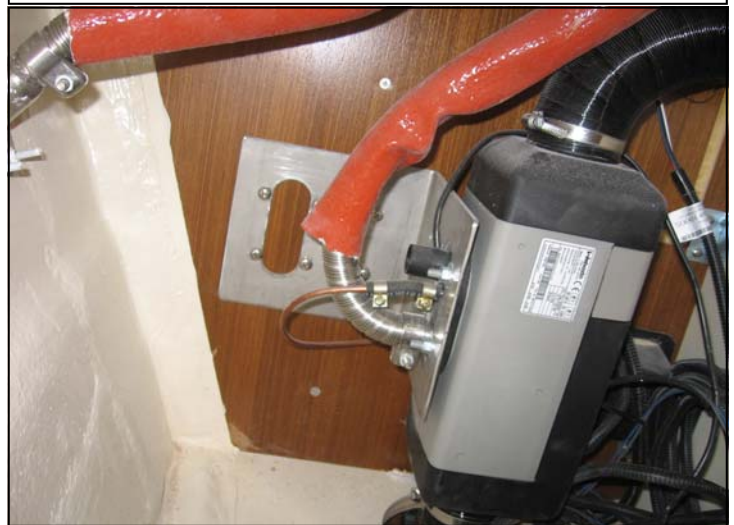
Heater unit is secured on L bracket, the unit locates inside aft cabin port euro shelf.
