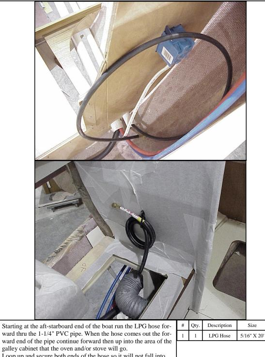
2. Loop up and secure both ends of the hose so it will not fall into the way when the module is placed into the hull.
