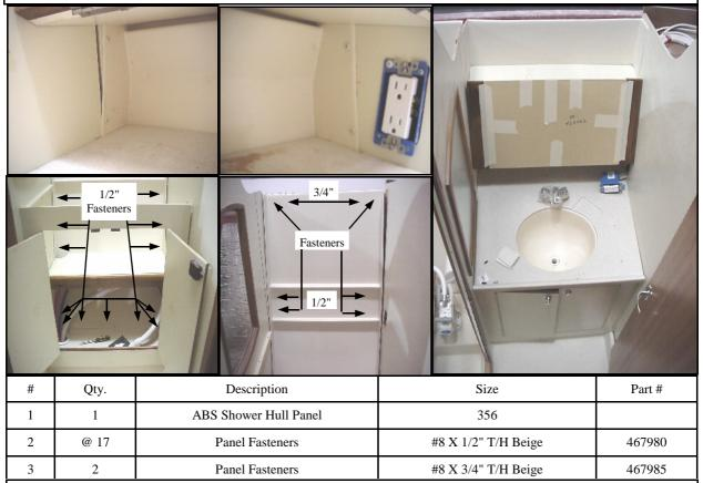
1. The vanity hull panel (28" wide, with two receivers) will be fastened to the bulkheads with truss head woodscrews.
