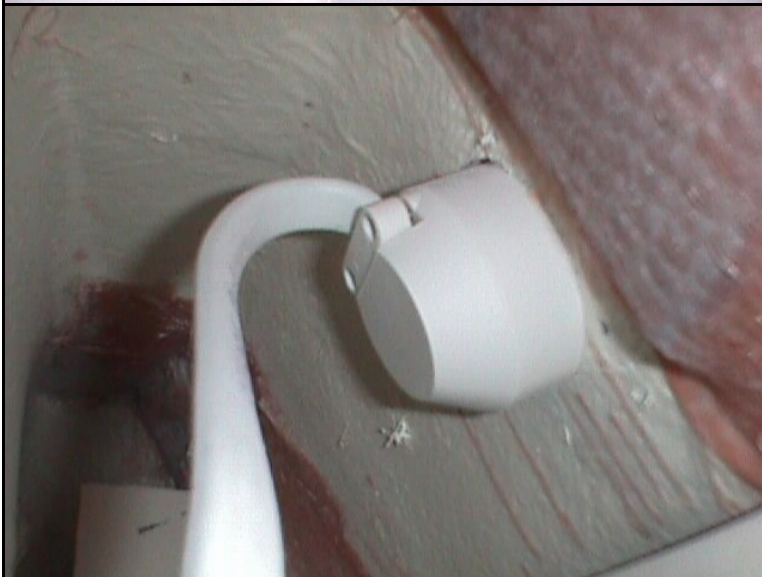
INSIDE VIEW OF SHORE POWER OUTLET AFTER IT HAS BEEN WIRED
