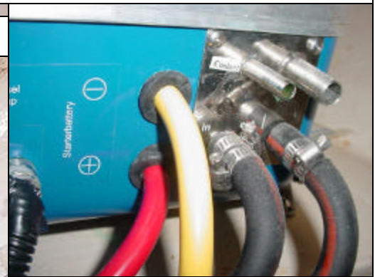
Fig 8. each fuel line requires 2 hose clamps for securing. Generator starter cable requires conduit.
