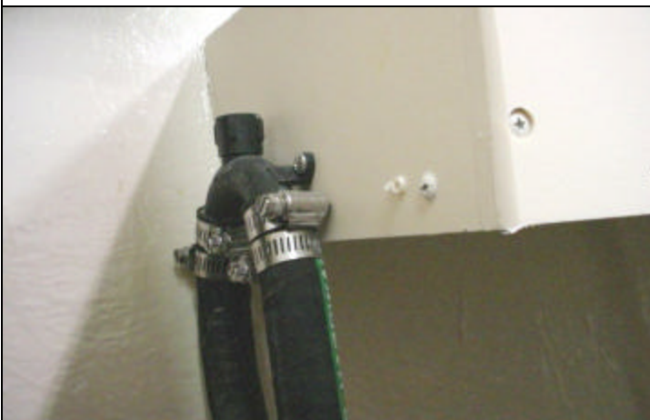
Fig 3. connect anti-siphon valve to vented loop coolant hoses then secure the valve on upper shelf.
