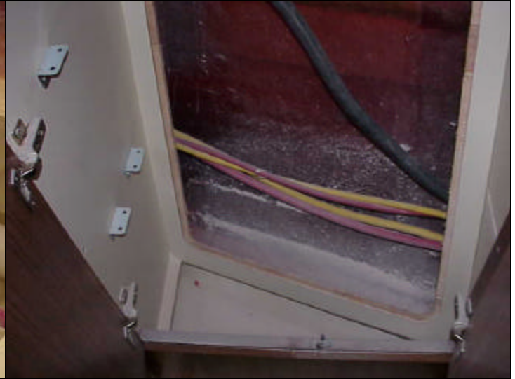
Cables continuing aft thru hanging locker.
