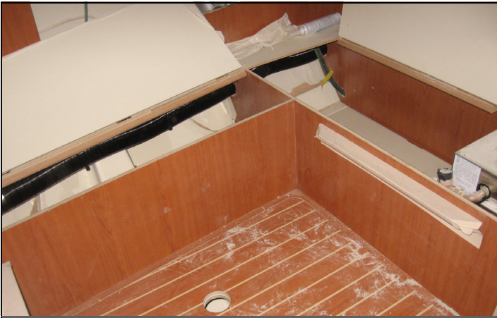
ø3.54" ducting comes out from galley area thru divider forward to fwd bunk
