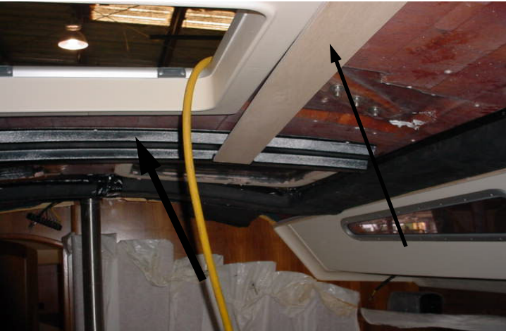
FIG 4. INSTALL CROSS AIR DUCT AND ANOTHER AIR DUCT IS LOCATE AT STBRD SIDE . INSTALL STBRD SIDE CENTER WHISPER GROUNDS
