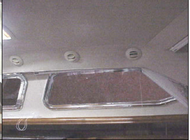
Main Cabin Port Side Forward Section Air Vents
