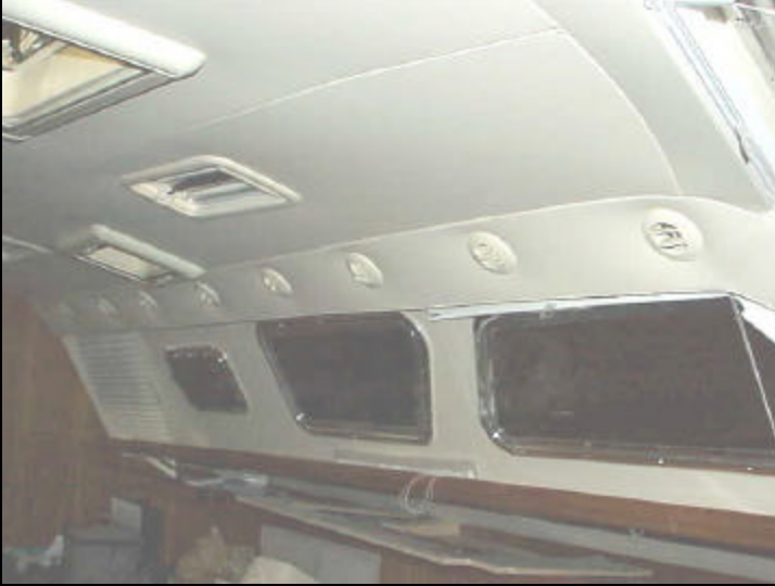
Main Cabin Port Side Air Vents ( 8 vents)
