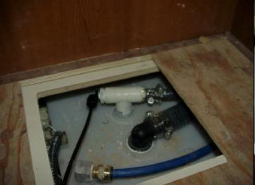
THE BRASS HOSE BARB FOR VENT HOSE ON WATER TANK WILL NEED TO BE REMOVED SO AN ALL THREAD TEE CAN BE INSTALLED. THE TUBE FROM THE "PRODUCT OUTLET" ON THE WATERMAKER WILL ATTACH TO THIS TEE. REATTACH THE BRASS BARB & VENT HOSE TO THE
