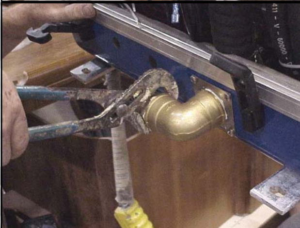
While the generator is in the air, attach the exhaust elbow and hose barb that come with the generator. Use pipe compound on the male threads and face the elbow towards the front of the generator.
