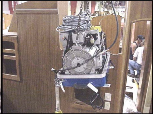
Using the center hoist lift the generator into the boat
