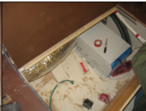
Run this air duct upward to chart electrical panel, install air duct to this air grill. The illustration shows on right hand indicating the ECU for fwd A/C unit & air grill.
