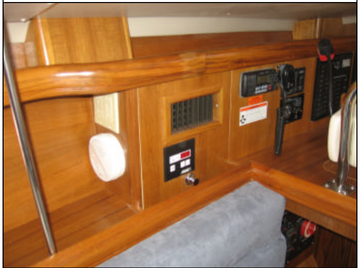
Complete installation of the ECU & Air vent on electrical panel .
