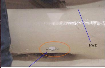
Follow bow thruster manual instruction to drill designated mounting holes for propeller drive unit.
