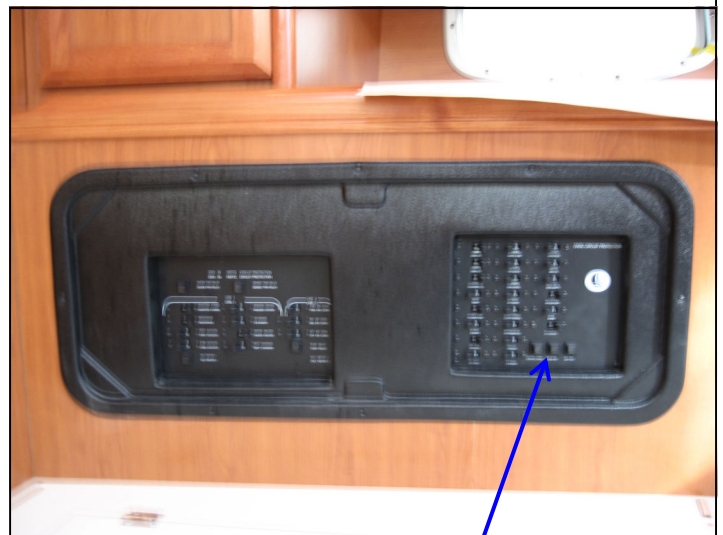
Get power supply from autopilot breaker
