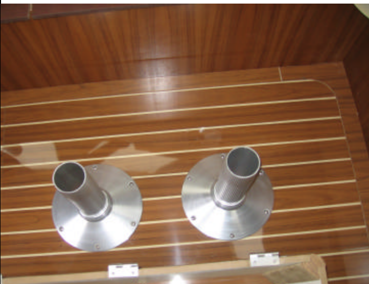
The illustration shows short columns were installed to floor bases
