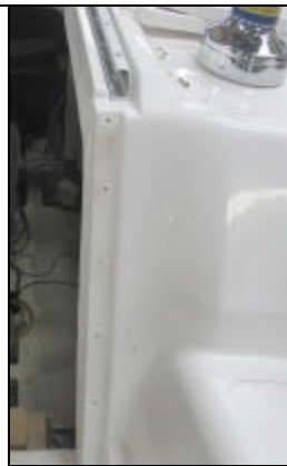
Drill mounting holes thru door frame
