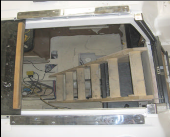
Overview of the slider & drop-in door installation
