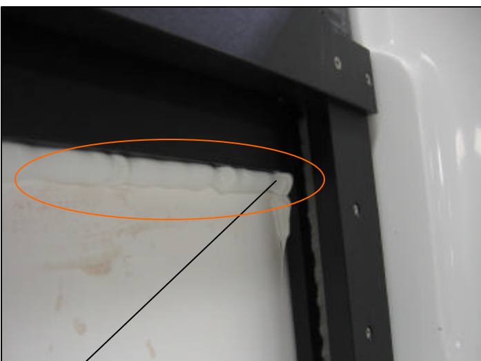
Door frame bottom edge caulking to close gap
