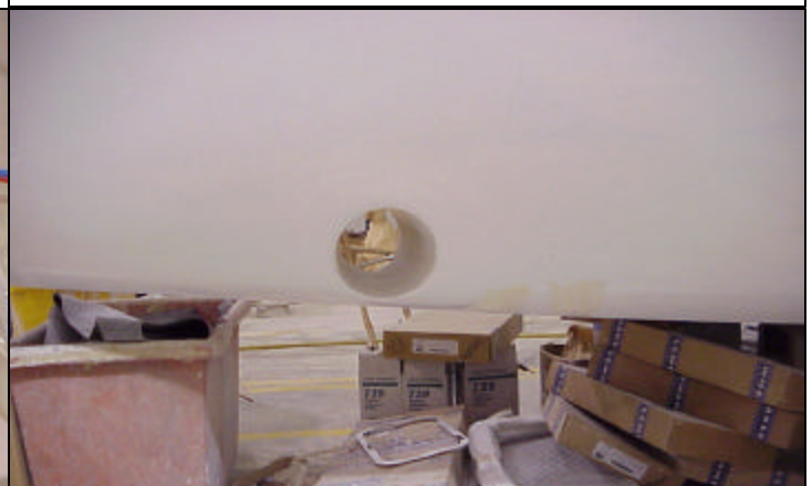
Grind 1" radius around outside edge of tube then gelcoat & buff
